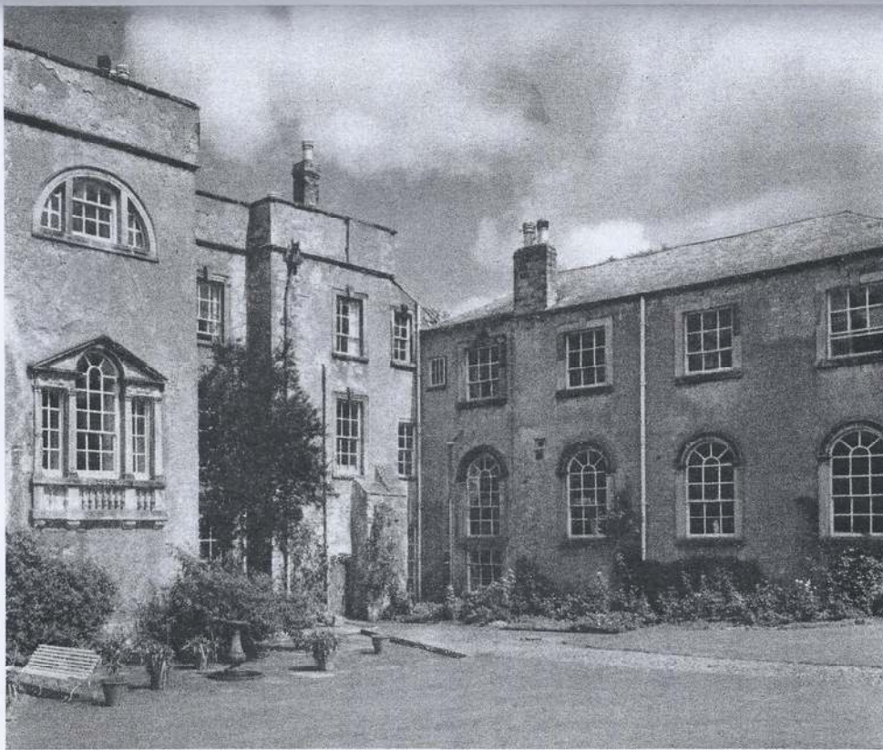
6.—PART OF THE SOUTH ELEVATION. The Venetian window lights the oak staircase, and the chapel wing lies on the right
